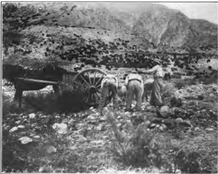
Convicts Collecting Stones for Crusher, Near Willard, Box Elder County.
